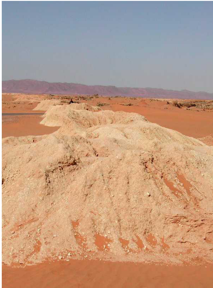
Fig 1– Drainage gallery seen at the surface: photo (Morocco)
